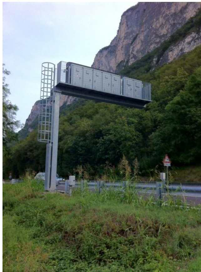
Figure 17: The Variable Message Sign in correspondence of which it was decided to activate the first static monitoring point.
