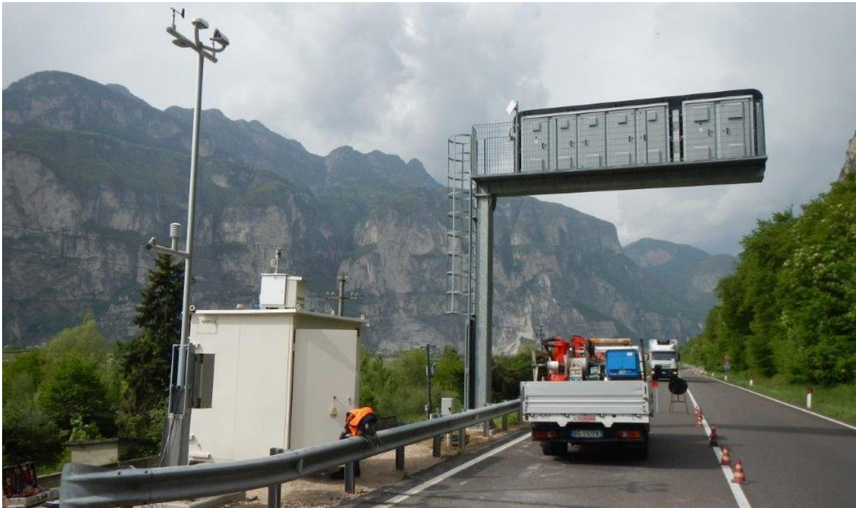
Figure 20: The road works organized during the installation of the first static monitoring site.
