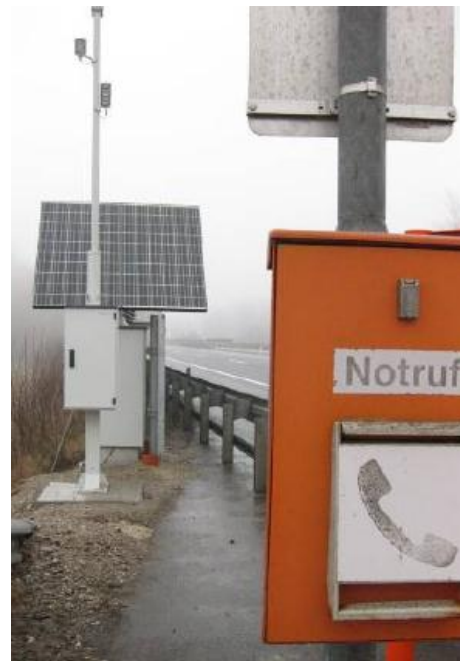
Figure 29: The fuel cell based power supply system installed within the ASFINAG highway network [48].
