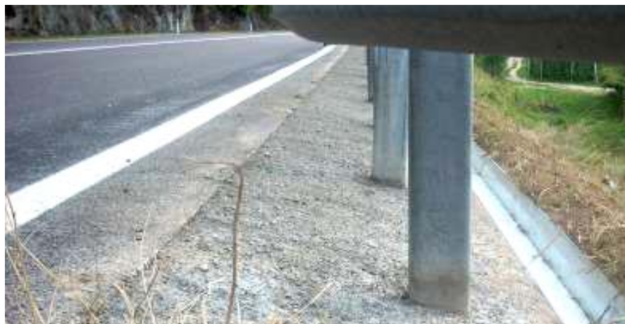
Figure 27: Runoff water collection and monitoring system - concrete gutters at roadside.
