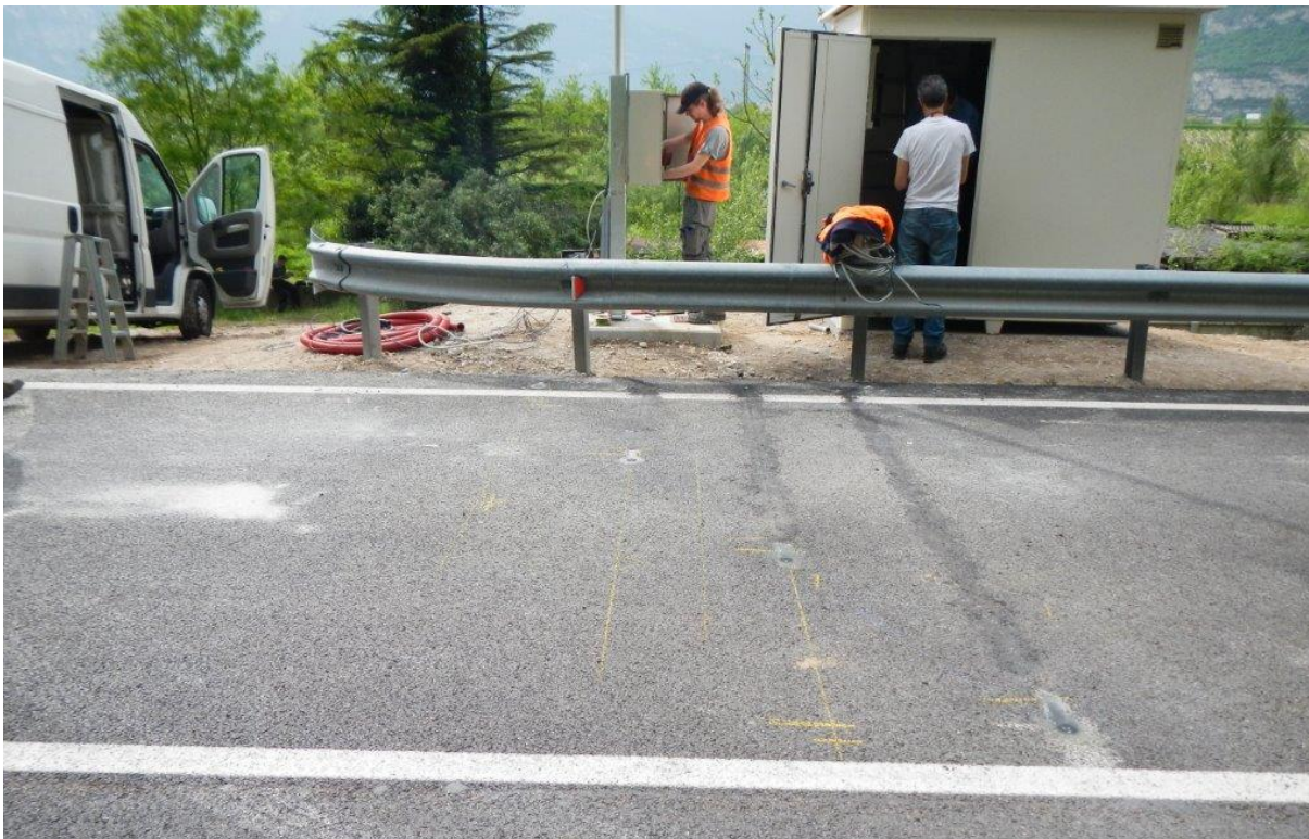
Figure 21: The positioning of the invasive sensors inside the road in correspondence of the first static monitoring site.
